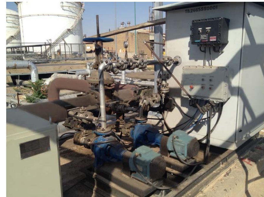
Auto Sampler System installed in Tabriz refinery
